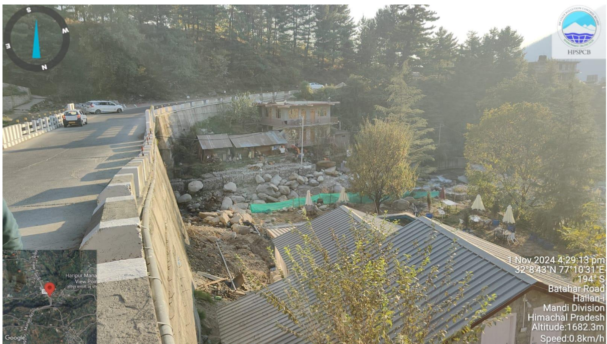
B). Haripur bridge open for vehicles on Haripur Nallah.
