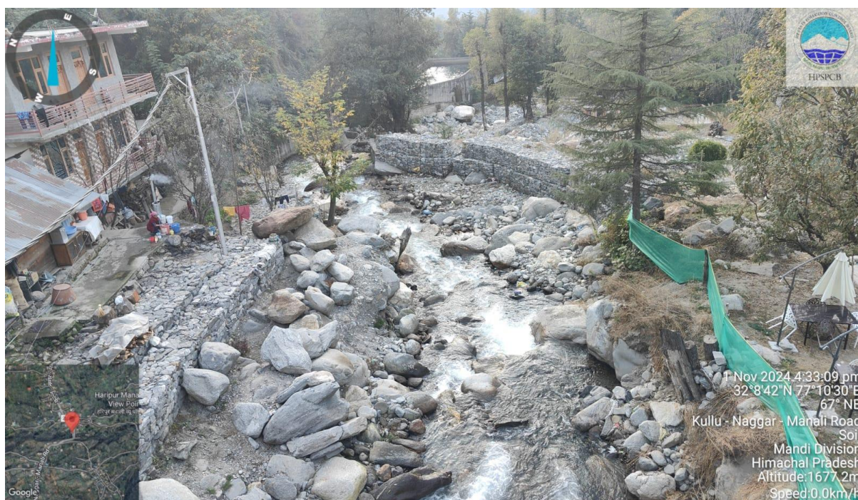
D). Crate walls provided downstream of Haripur bridge towards the fish farm and of opposite side.
